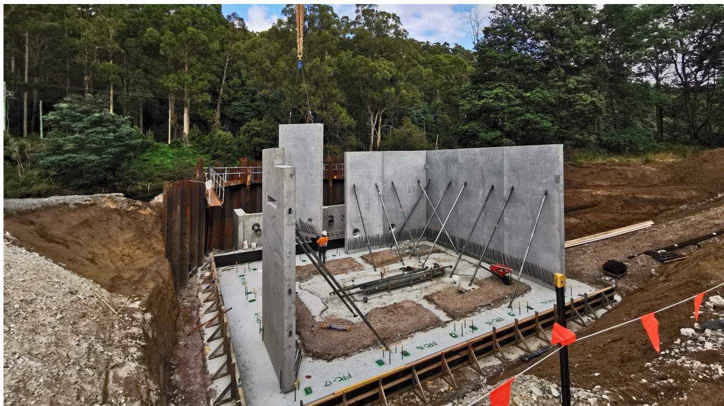
Precast panel installation at Forth pump station on the Don Irrigation Scheme
