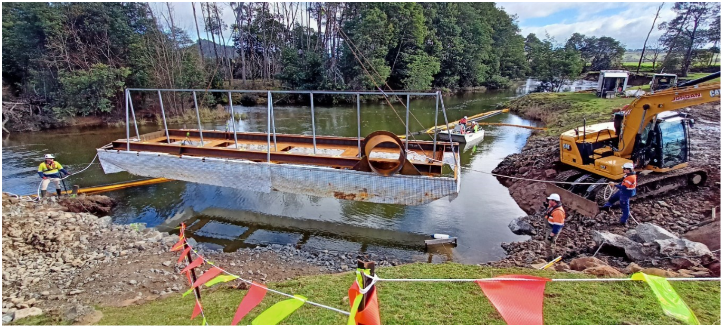
Intake screen formwork installation at Quamby
